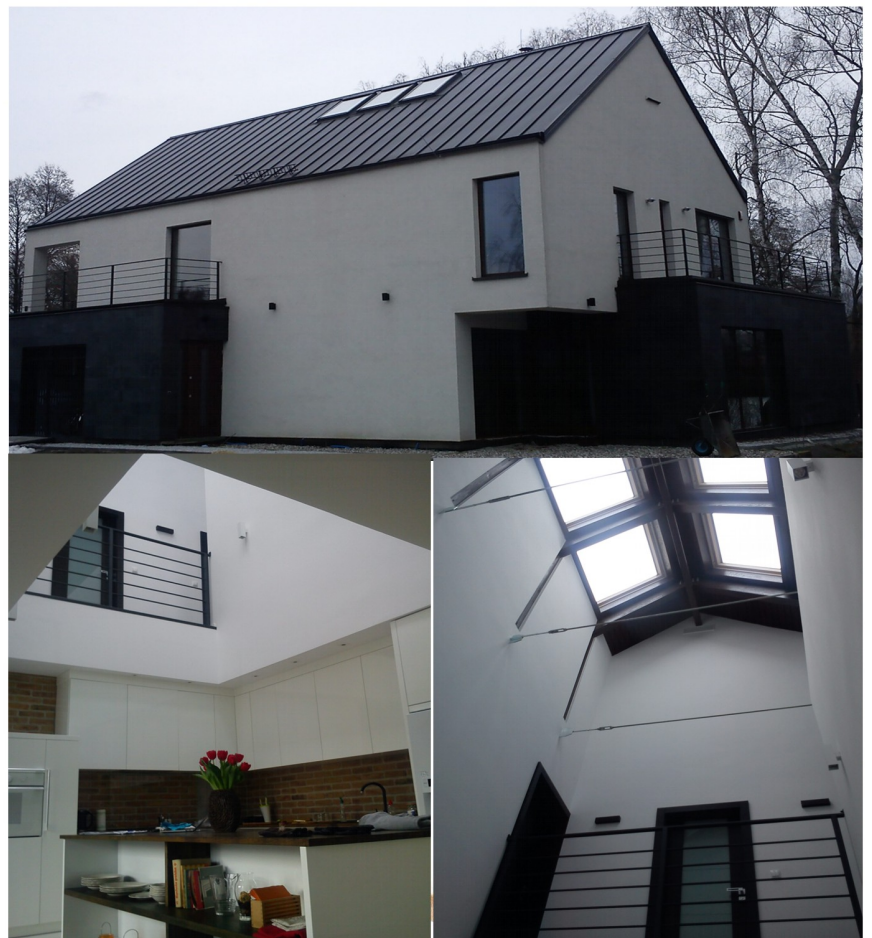
Fig. 4. Image of the designed Tuscan style home, currently under construction on a site near Warsaw incorporating saw-tooth skylight allowing natural light to all the floors.
