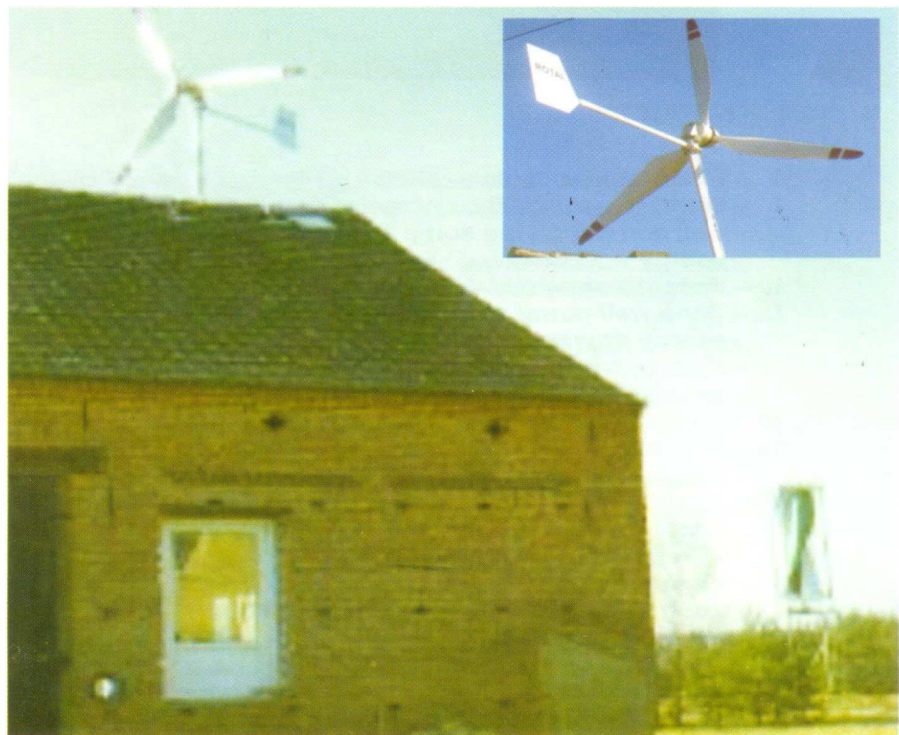
Fig. 5. Horizontal axis wind turbine, 3.5 kW nominal capacity.
